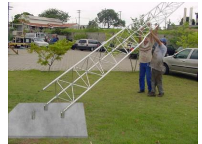
Swivel mounting supports for easy installation and maintenance
